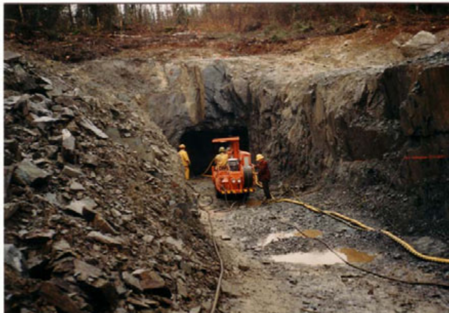
Figure 6.1 – Decline ramp excavated on the Flordin property
