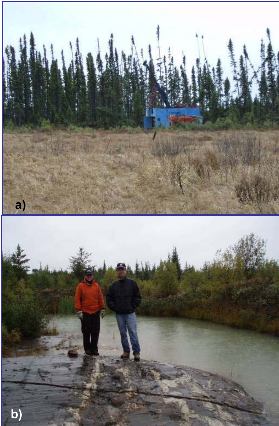
Figure 14.1: a) Diamond drilling on the Discovery Project; b) Quartz-ankerite mineralized shear zone still exposed at the Discovery stripped zone (Zone B, October 2006)
